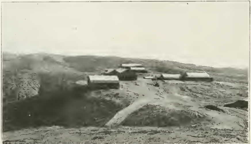
Plate I. General layout of Pacific Oil Company Camp in Elk Hills District, Kern County, California. This camp illustrates what can be done at relative small cost for the welfare of the men.
